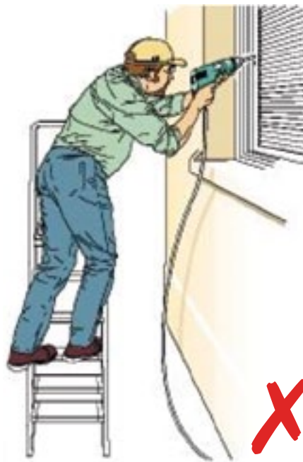
Figure 31: Incorrect – steps are side-on to work activity.
