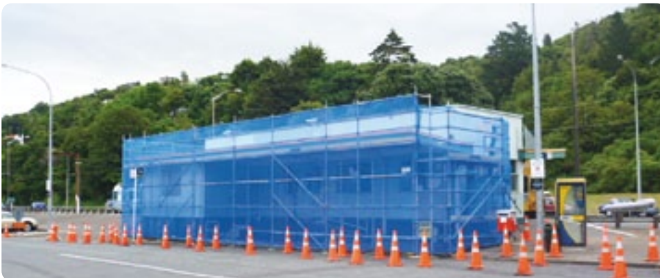
Figure 3: Covered scaffolding on a single storey building.
