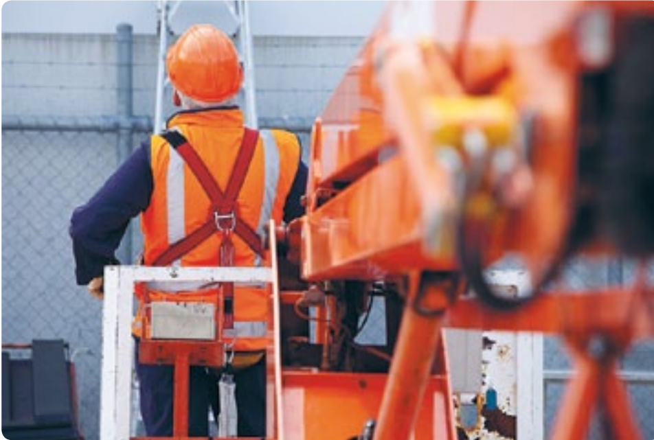
Figure 1: A worker restrained in boom-style elevating work platform (EWP).
