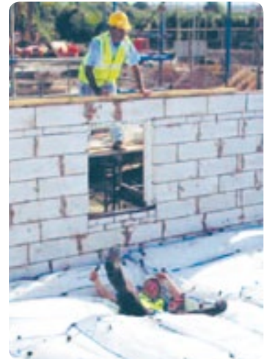
Figure 27: A worker falls into a soft landing system.
