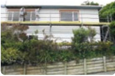
Figure 4: Scaffolding on a residential building.
