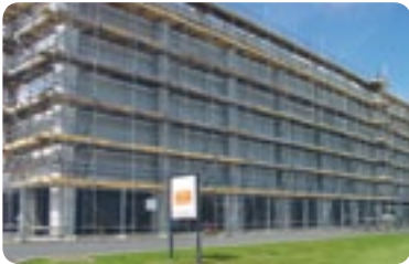
Figure 5: Scaffolding on a multi-storey building.
