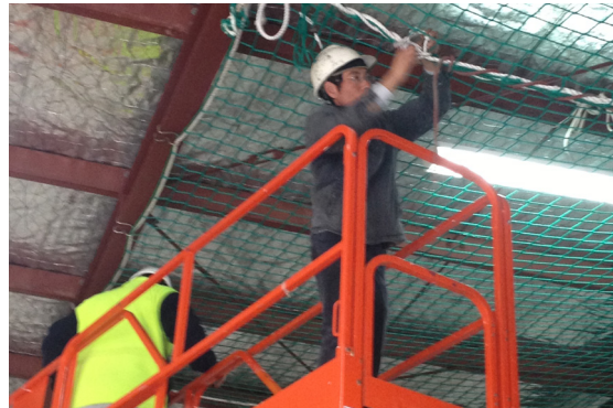
Figure 14: Dismantling safety nets.
