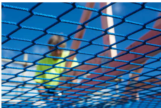
Figure 1: Knotless, square mesh safety net.
