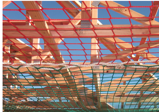
Figure 13: Safety nets joined by lacing.
