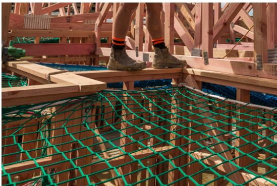
Figure 6: Safety net with between 5-10% initial sag.
